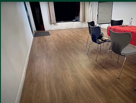
New floor for a local community facility
