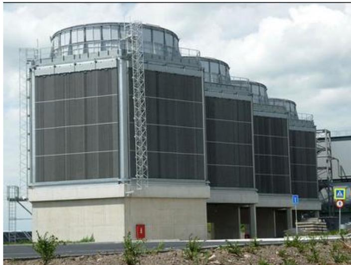
**Figure 9: ACC Installation example (1) Figure 10: ACC Installation example (2)**
