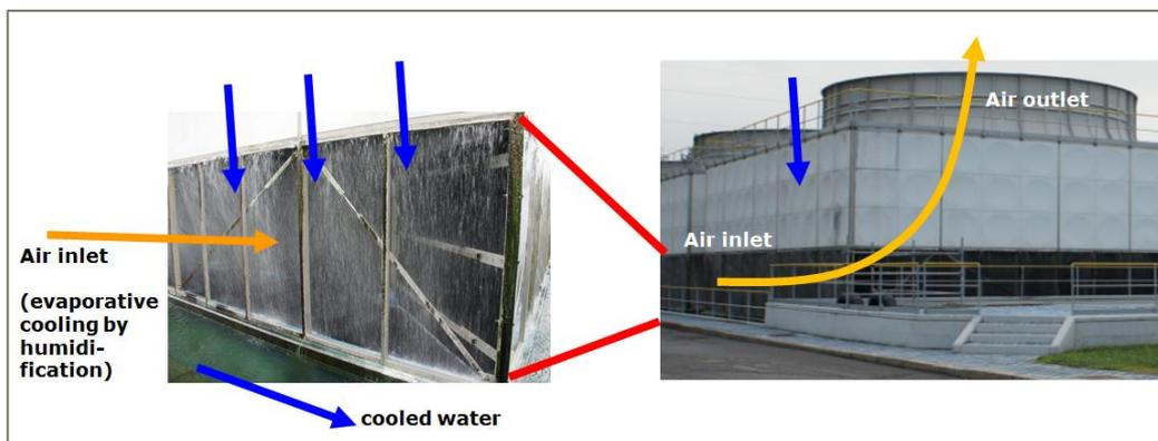
Figure 15: Pictures and principles of cooling tower
