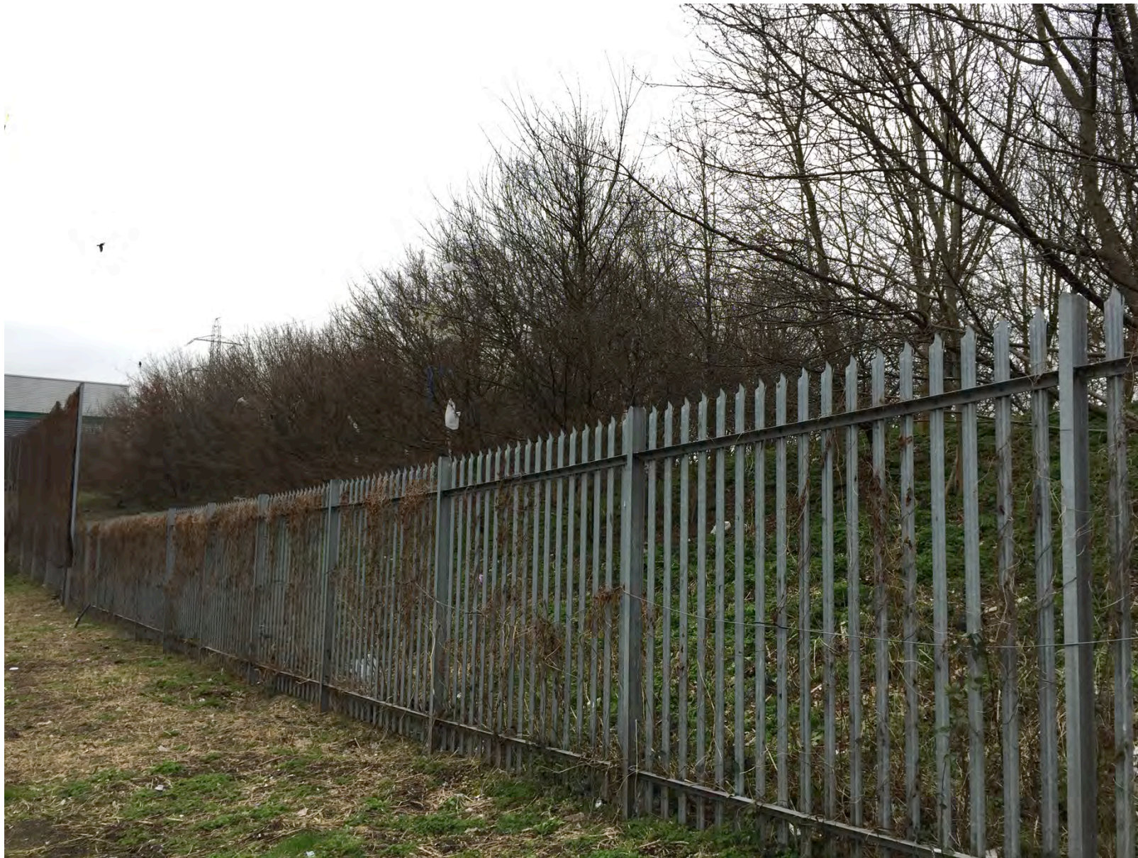
Photograph 17: Looking North-east into Group 16
