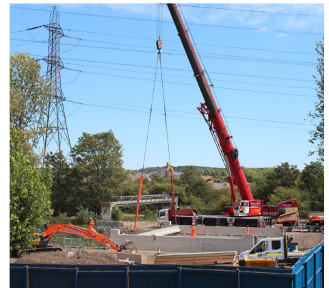
Beams and bridge being installed over the Enfield Ditch to form a new eastern access into the EcoPark
