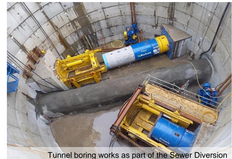
Tunnel Boring Machines used at the Sewer Diversion site
