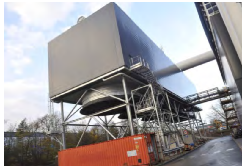
Figure 6.123: Example of a cooling condenser
