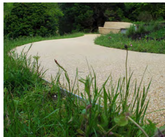
Figure 6.102: Resin bound gravel footpath
