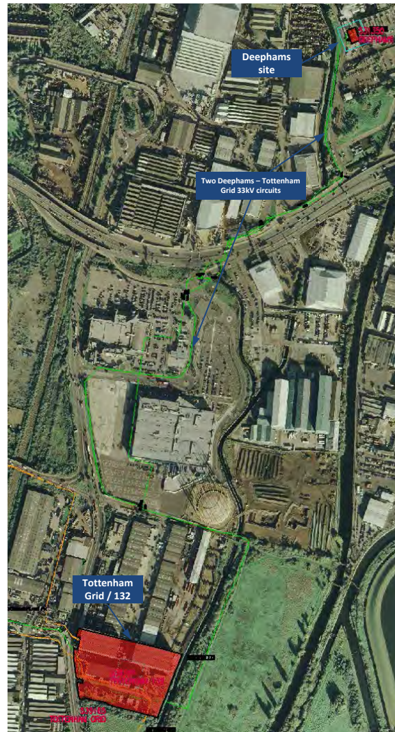
Figure 4 - Aerial view of the Deephams connection at present
