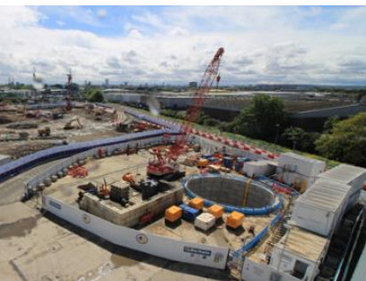
Sept 2021: Completion of the Sewer Diversion
