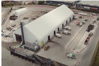
April 2022: Completion of the Temporary Bulky Waste Recycling Facility
