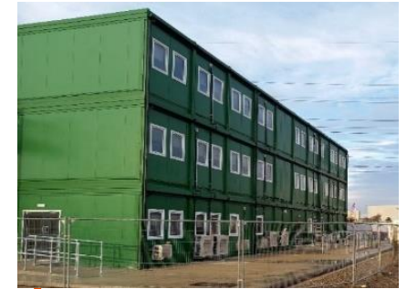
March 2021: Construction of the Laydown Area offices
