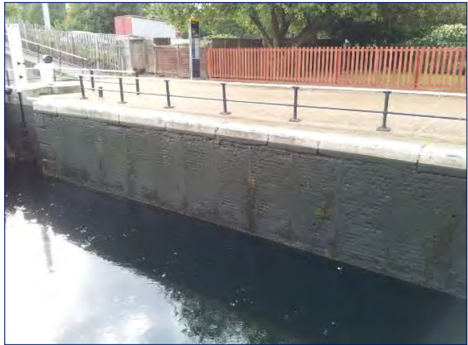
Figure 5-5: Typical lock wall condition (Tottenham)
