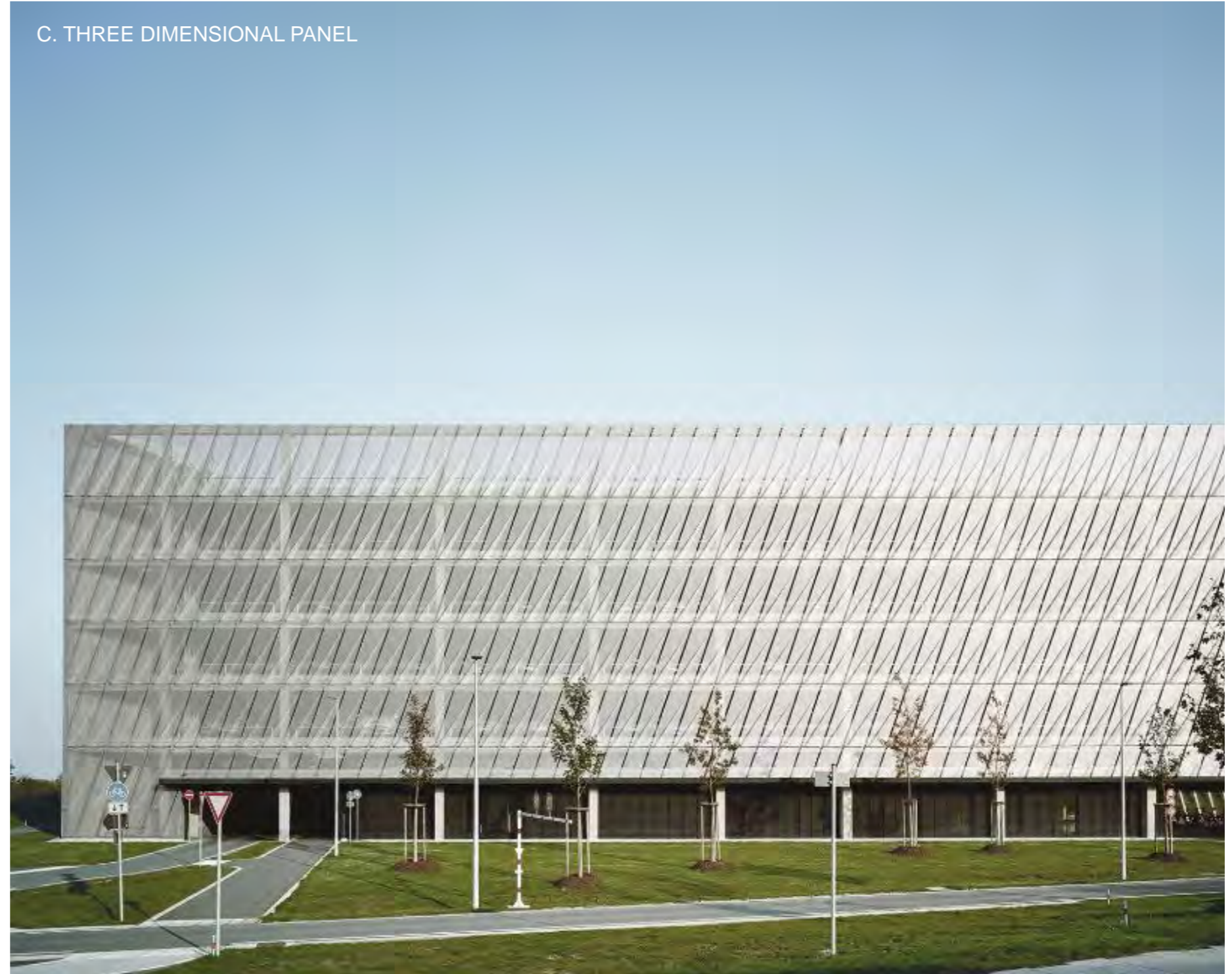
Figure 6.56: Existing example of three dimensional panels: Adidas Parkhaus, Germany
