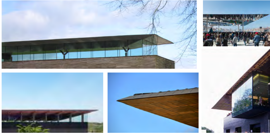
Cantilevered 'Feature Roof' examples
