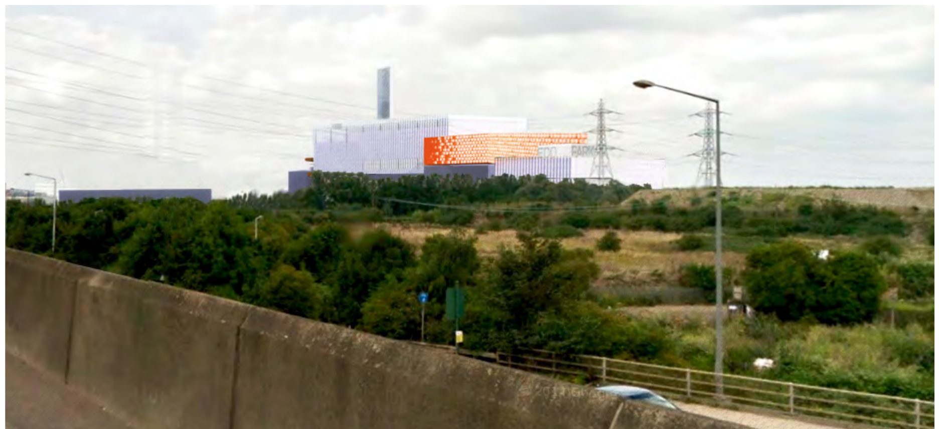
Figure 6.83: Illustrative view from A406 North Circular Road, east. Accent colour on crane hall provides contrast between process hall and tipping hall volumes.
