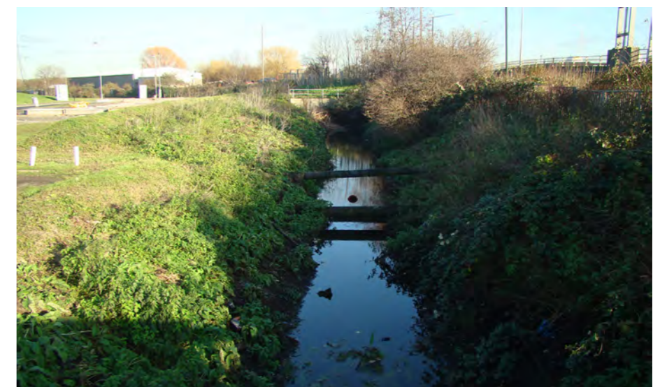
Figure 4.20: Enfield Ditch, along the southern edge of the Application Site
