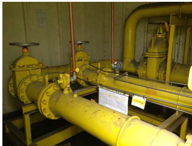
Figure 2.2: Detail of the pressure reduction system – angle 2
