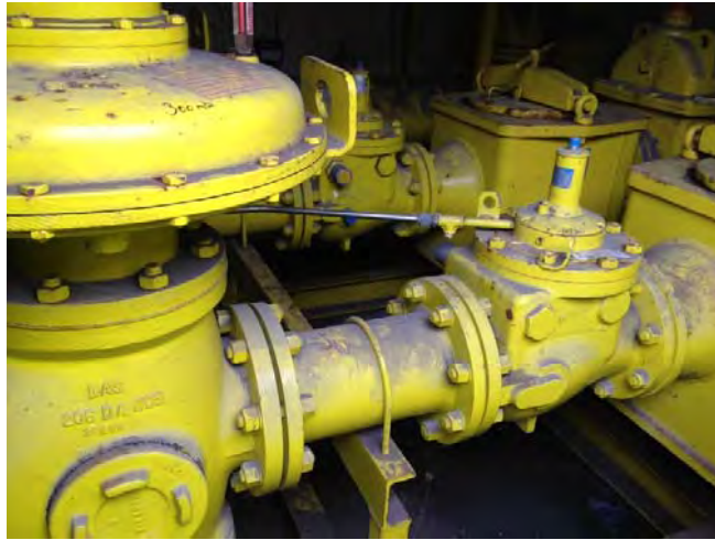
Figure 2.1: Detail of the pressure reduction system – angle 1
